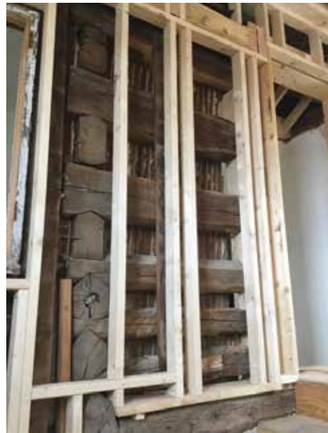
LEFT: The northwest corner of the original cabin showing its construction method and hand-yewn logs.
