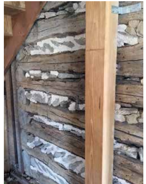
LEFT: The northwest corner of the original cabin showing its construction method and hand-yewn logs.
